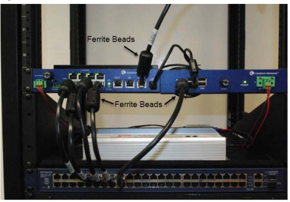
Figure 34: Ferrite Beads on a USB Cable
