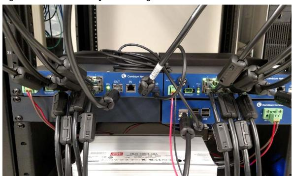
Figure 19: Controller to Injector Cabling
