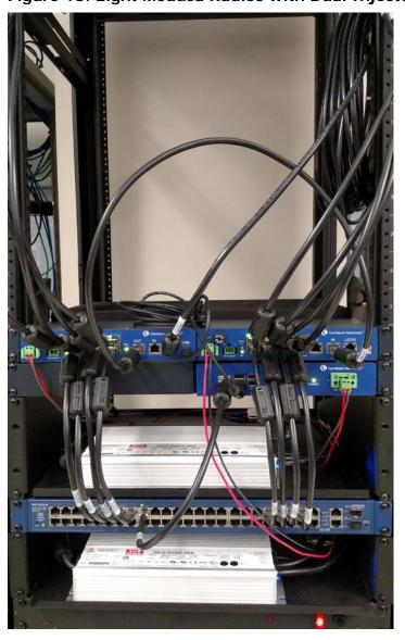
Figure 18: Eight Medusa Radios with Dual Injectors
